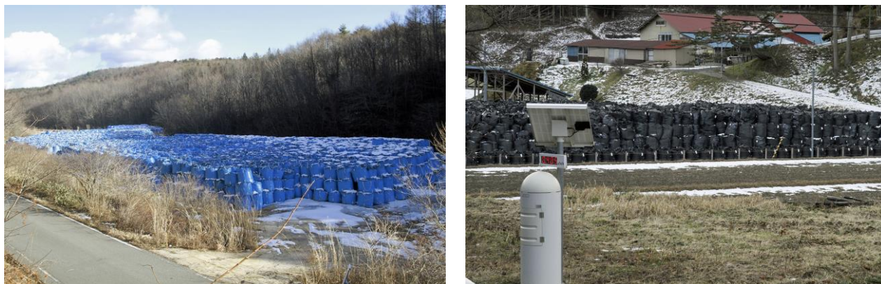
Figure 1.12: After decontamination work, resulting radioactive waste is packed into flexible containers. The containers are then stacked in layers in rice paddies, road sides and empty lands. They are also buried beneath private lands and school yards. Radiation dose in these areas is high. (Radioactive waste temporarily stored in Kawauchi Village and Miyakoji District in Tamura City. Photos taken by Shinya Sato on 6 January 2016.)
